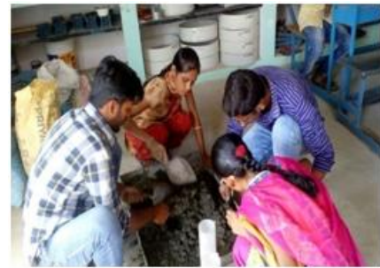
Fig Mixing of concrete
