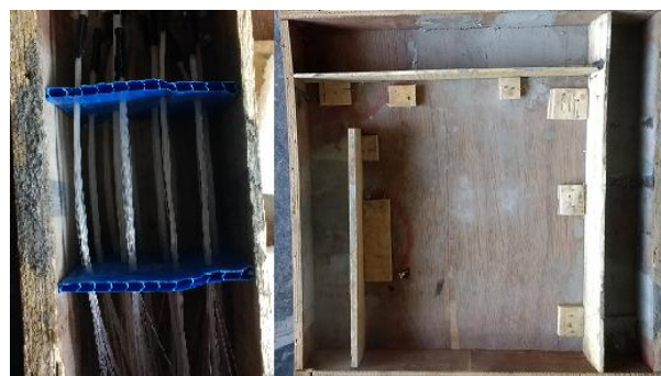
Fig 19: MAKING OF WODDEN MOULDS FOR OPTICAL FIBER CUBES.
