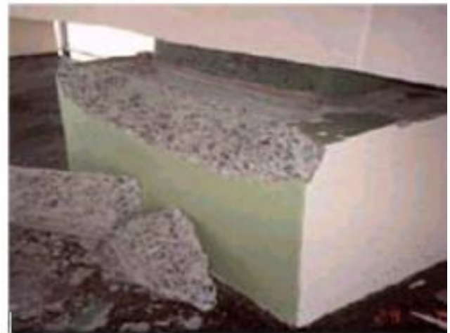
Figure 10. Damaged concrete pedestals of the elastomeric bearing of the New Surajbadi Highway Bridge.
