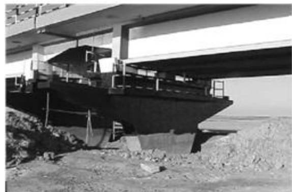
Figure 8. Girder-pier support system on the Well foundation bearings of the New Surajbadi Highway Bridge. is not visible.
