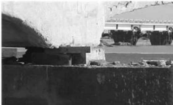
Figure 6. Damaged bearing on Old Surajbadi abutment of the Old Surajbadi Highway Bridge.
