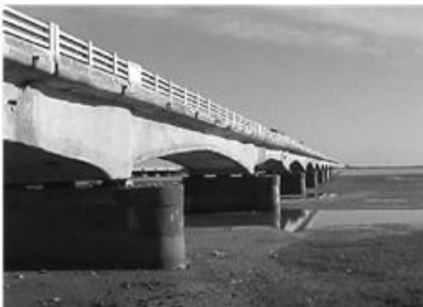
Figure 3. Old Surajbadi Highway Bridge
