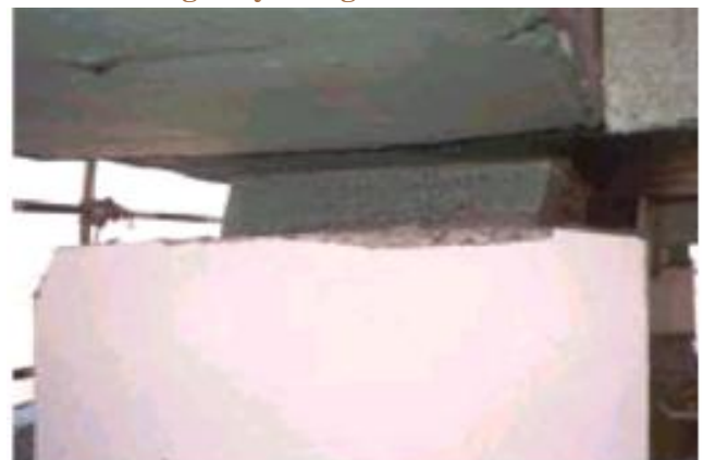
Figure 9. Severely strained elastomeric New Surajbadi Highway Bridge.
