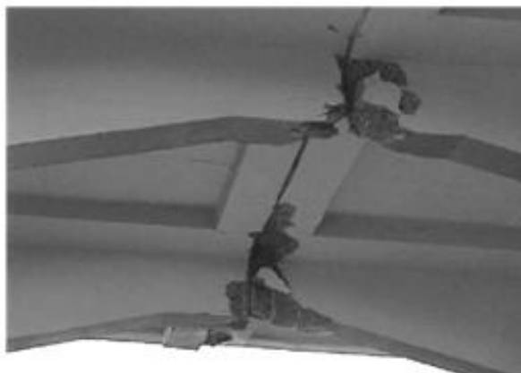
Figure 13. Pounding between two adjacent superstructure decks of the New Surajbadi bridge spans, Highway Bridge.
