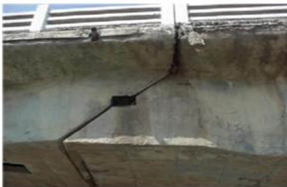
Figure 7. Failure of in-span hinge and traffic railings at Old Surajbadi Highway Bridge.
