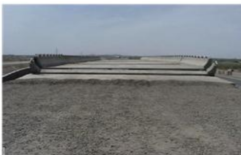
Figure 16. Failure of approach slab of a bridge at the village Vondh.
