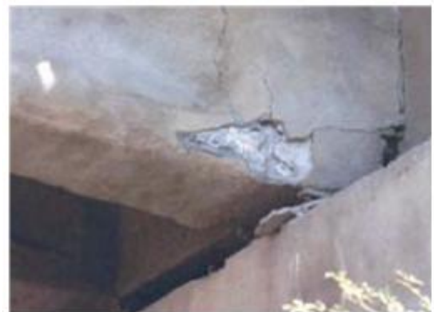
Figure 11. Damaged soffit of the girder at the span ends of the New Surajbadi Highway Bridge.
