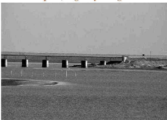
Figure 14. Near the south side abutment of the Surajbadi Railway Bridge.
