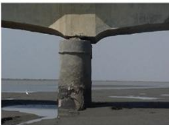
Figure 4. Relative longitudinal movement between the piers and the superstructure spans in the Old Surajbadi Highway Bridge.
