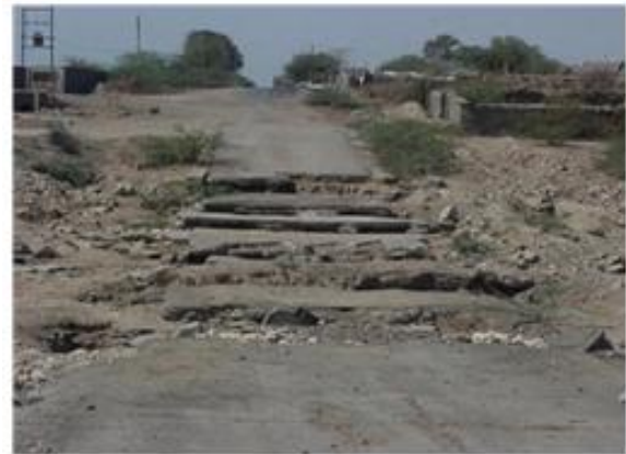
Figure 2: Collapse of structure between towns of Anjar and Bhuj.
