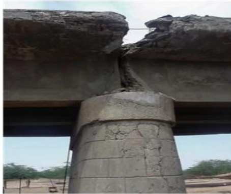
Figure 15. Failure of the girder end and expansion joint of a bridge between the towns of Gandhidham and Bhachau.
