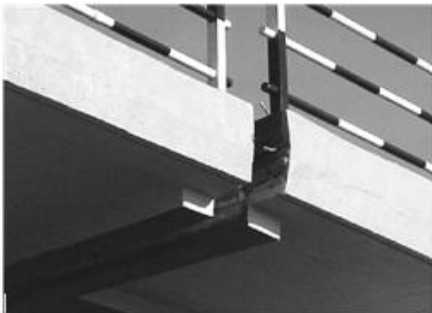
Figure 12. Transverse displacement of the New Surajbadi Highway Bridge.
