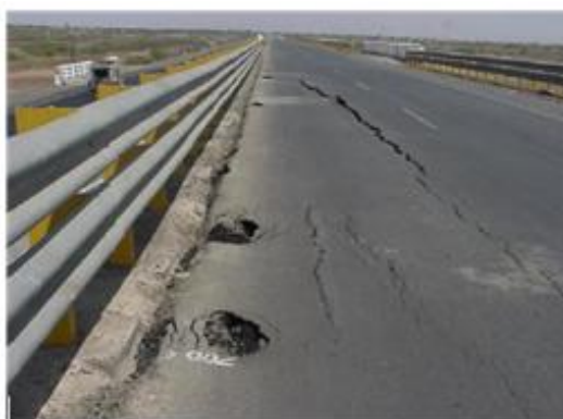
Figure 1: Roadway cracking between the roadway drainage towns of Gandhidham and Bhachau.
