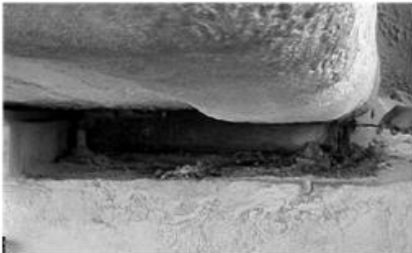
Figure 5. Roller bearing on the north side
