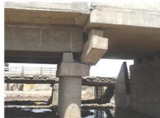
Figure 17. Failure of crossbeam of a bridge at the village Vondh.
