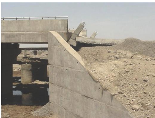
Figure 18. Failure of abutment of the bridge at the village Vondh.
