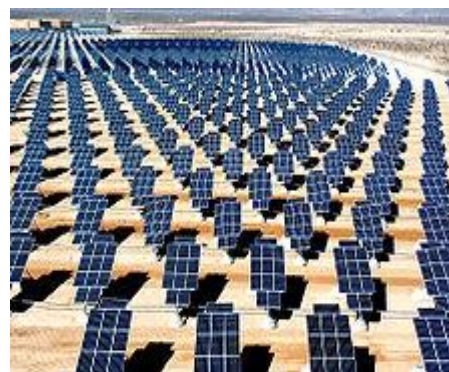
Fig.2 Photovoltaic power station,.
