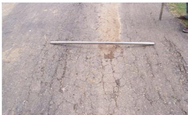
Figure 1 shows atypical cracking pattern PWD Singaram Stretch
