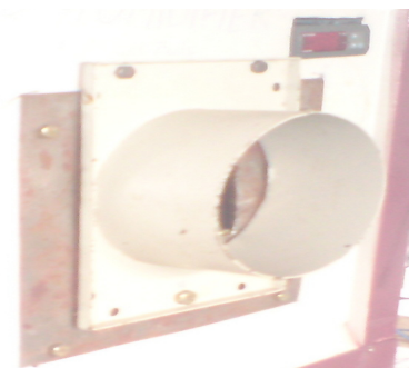
Figure 9: Image of Wind Outlet
