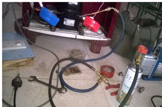
Figure 4.5: Refrigerator set up when Gas Charging of HC Mixture
