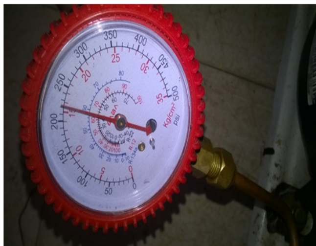
Figure 4.2: Discharge Pressure gauge
