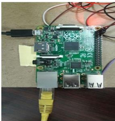
Fig. Fire sensor and raspberry pi hardware implementation
