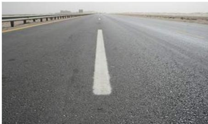
Figure 1 Typical Two-Lane, Two-Way Highway (Picture Courtesy of FHWA)
