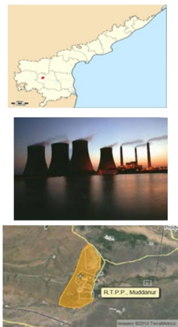
Fig 1: Rayalaseema thermal power plant – location map
