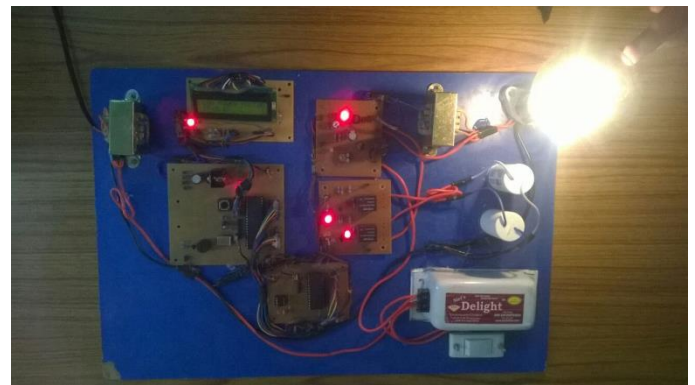
Figure 4: Practical observations before switching ON the capacitor
