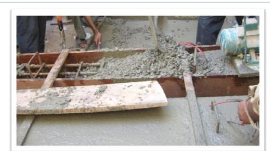
Fig.4.6.1 Casting of Beam Specimen
