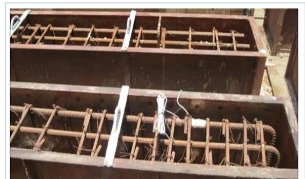
**Fig.4.2.1 (b) Steel Formwork**
