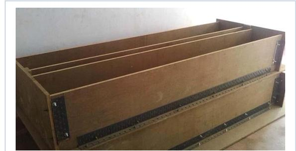
**Fig.4.2.1 (a) Wooden Formwork**
