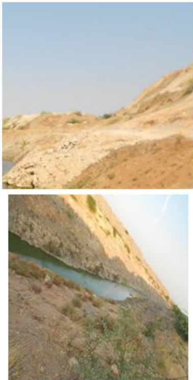
Somasila Reservoir back water
