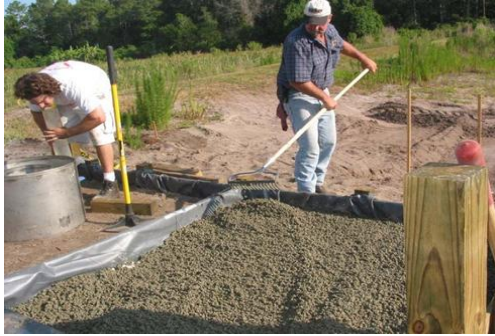
Figure 3: Stormwater Academy Porous Concrete Test Cell Installation
