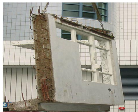
Figure2.4 Protocol of finished lightweight concrete precast wall
