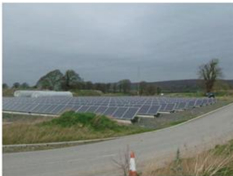
Fig. Ground Mounted Solar Array
