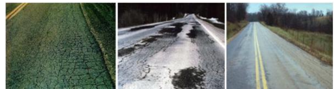
Fig 4.2- Fatigue cracking
