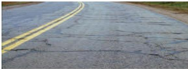
Fig 4.4 block cracking
