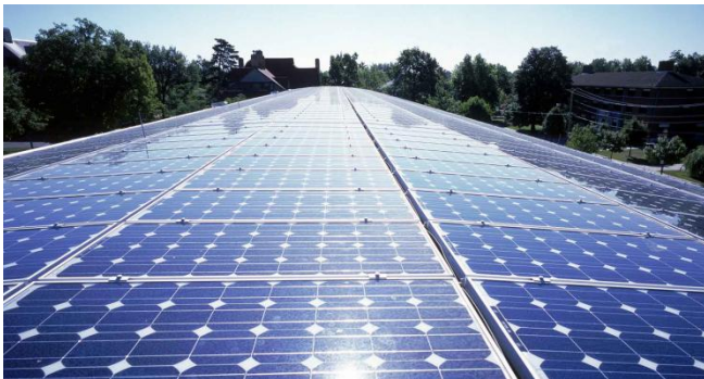
A large silicon solar array installed on the roof of a commercial building.
