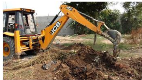
Fig.1.1. Earth digging operation
