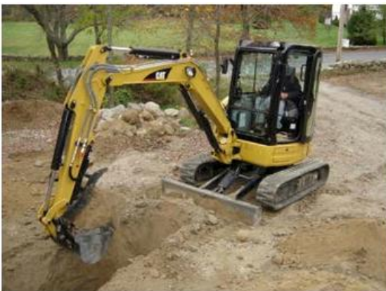
Fig 1.3: Trenching operation
