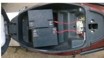
Fig .Arrangement of Batteries
