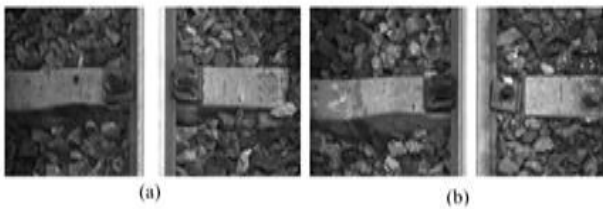
Worn and missing fasteners.
