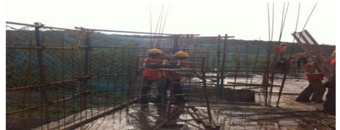
Figure 6.3 Safety ropes provided at edges Full Decking of Openings
