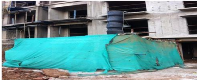
Figure 4.2 Debris Chute for Controlling Dust
