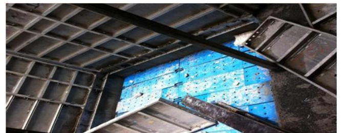
Figure 6.4 full decking of openings
