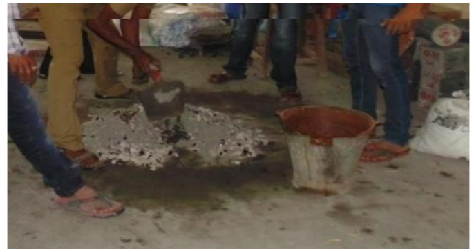
Fig 4.4: Mixing of concrete ingredients
