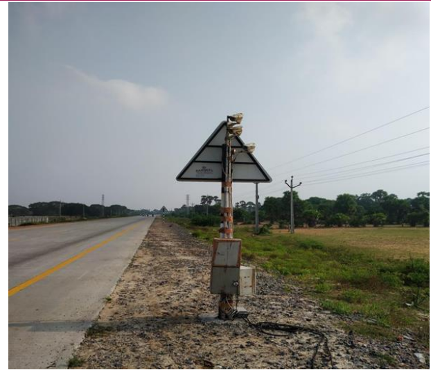
FIGURE.6 Pneumatic tubes for data collection though CC camera
