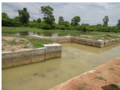
Fig (Inlet weir)
