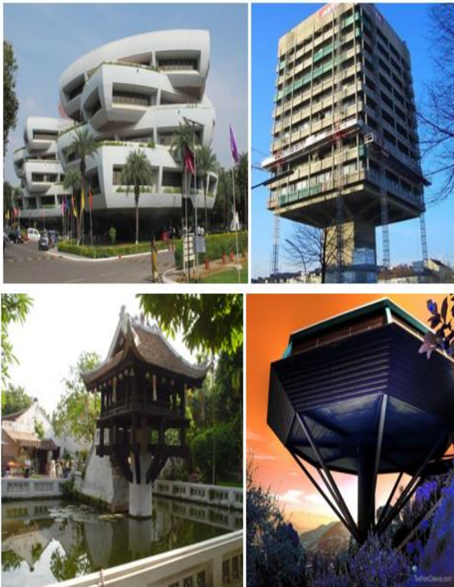
Fig.1.1: Structures supported on single column
