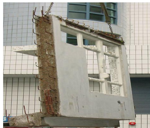
Figure 2.4 Protocol of finished lightweight concrete precast wall
