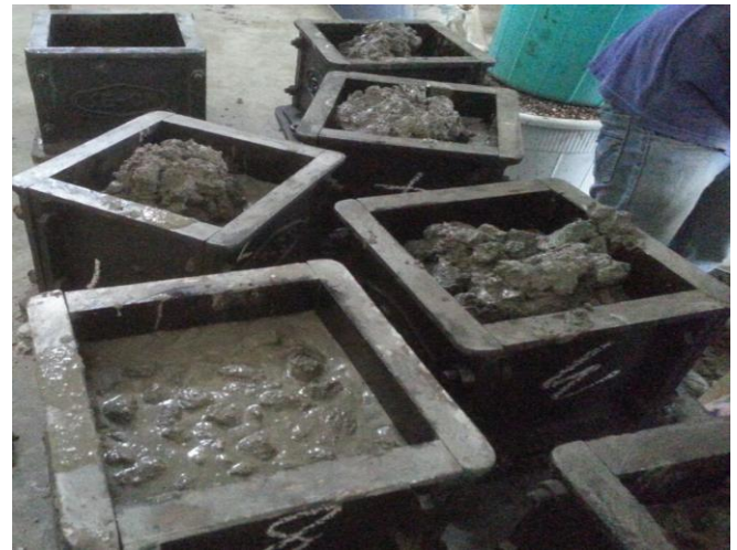
Fig 4.3 Casting of concrete
