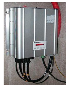
Inverter for grid connected PV
