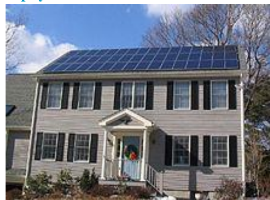
A 5.3 kW residential rooftop system near Boston, United States.
