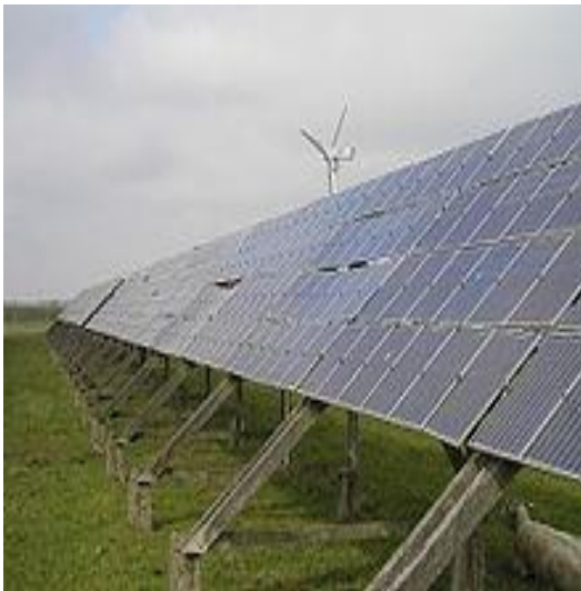
A 23-year old, ground mounted PV system on a North Frisian Island, Germany
