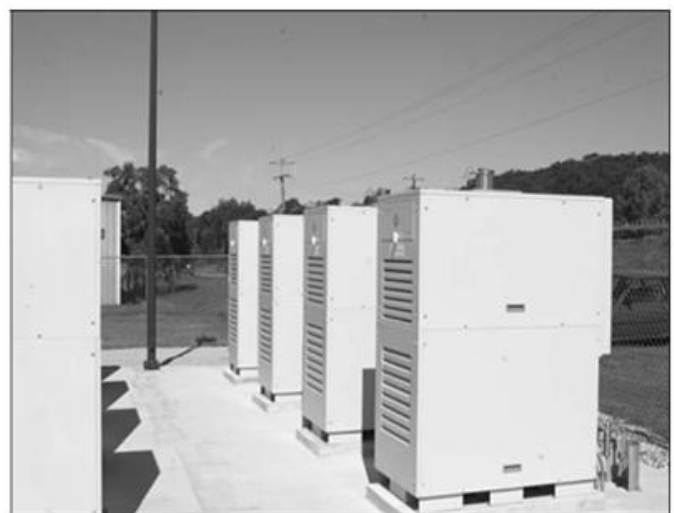
Fig.3.4 Capstone Microturbine, 30Kw
