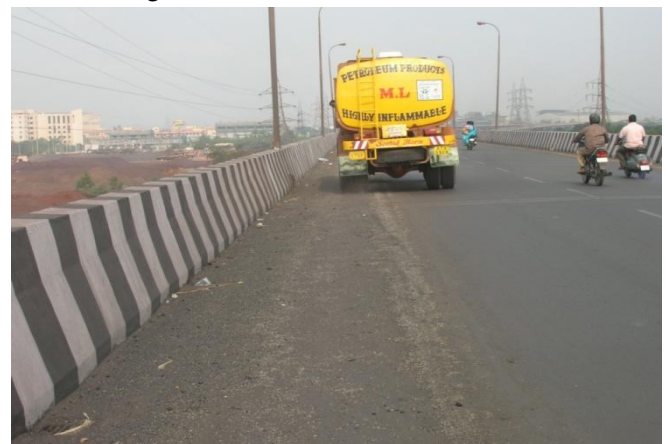
Fig.4. A typical screening site on which MS2D loop probe survey was done in Visakhapatnam city national highway on the road corridor
