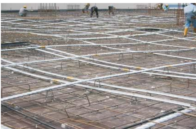
FIG6: SHOWS THE TENDON LAYOUT READY FOR THE CONCRETING.
