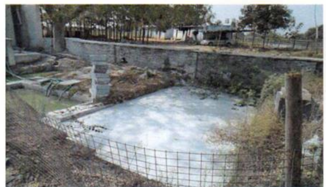
TSP Powder Slurry Storage Tank
