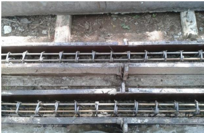
FIG 4.2. Beams formwork
