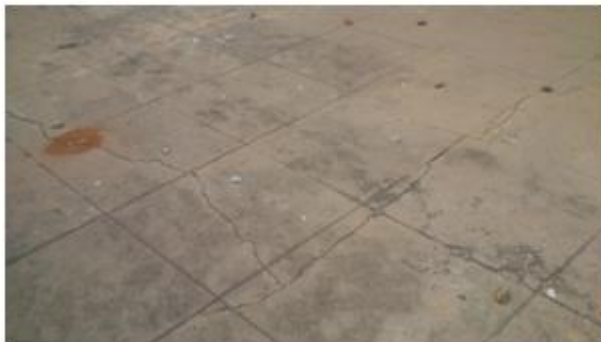
Fig 4 Cracks in concrete slab due to drying shrinkage
