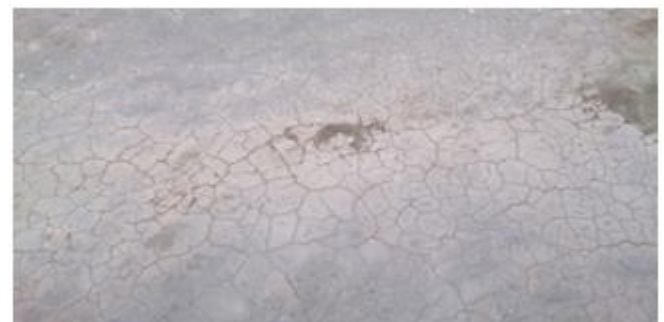
Fig.5 Cracks due to crazing
