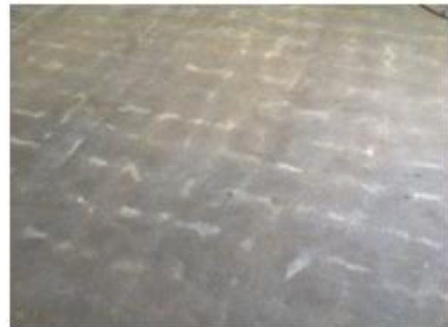
Fig 1: Cracks in concrete due to plastic settlement
