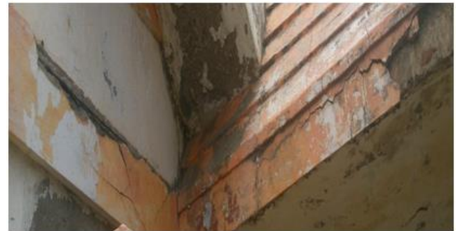
Fig.6 Beam: corrosion destruction of concrete cover; due to the longitudinal and transversal steel reinforcements by chloride attack
