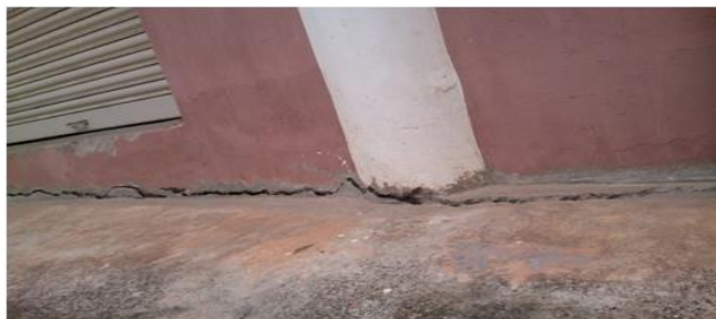
Fig.8 Crack is structure due to non uniform settlement of ground
