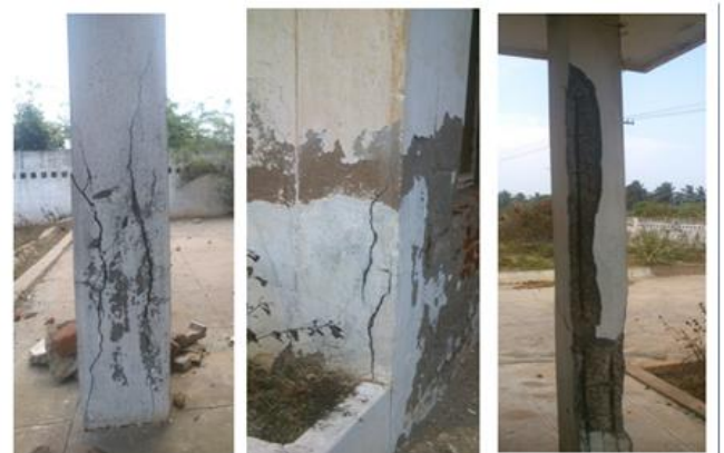
Fig.7 cracks in column due to corrosion of reinforcement in column
