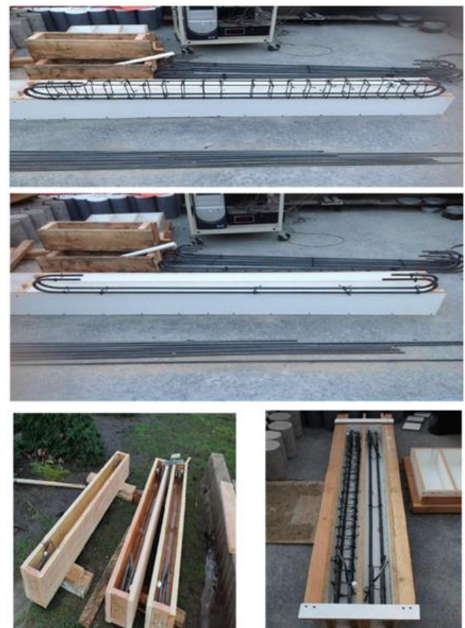
Figure 3-4 Steel fabrication and form work
