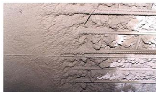
Fig 1.2: concreting of fire damaged slab
