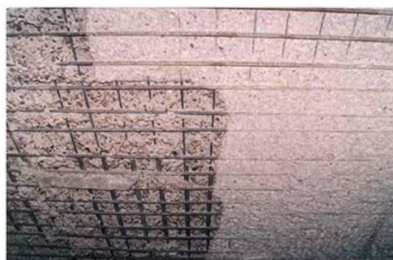
Fig 1.1: fire damaged slab
