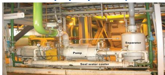
Fig5.1: Vacuum pump setup in industry
