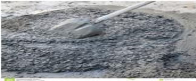
Fig-2.4 Concrete mixing
